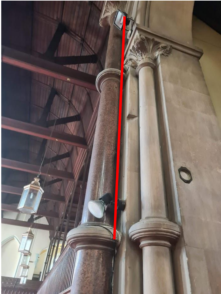
CABLE FOLLOWS DETAIL IN THE CORNER AND EXISTING CABLES FOR MOST THE RUN
