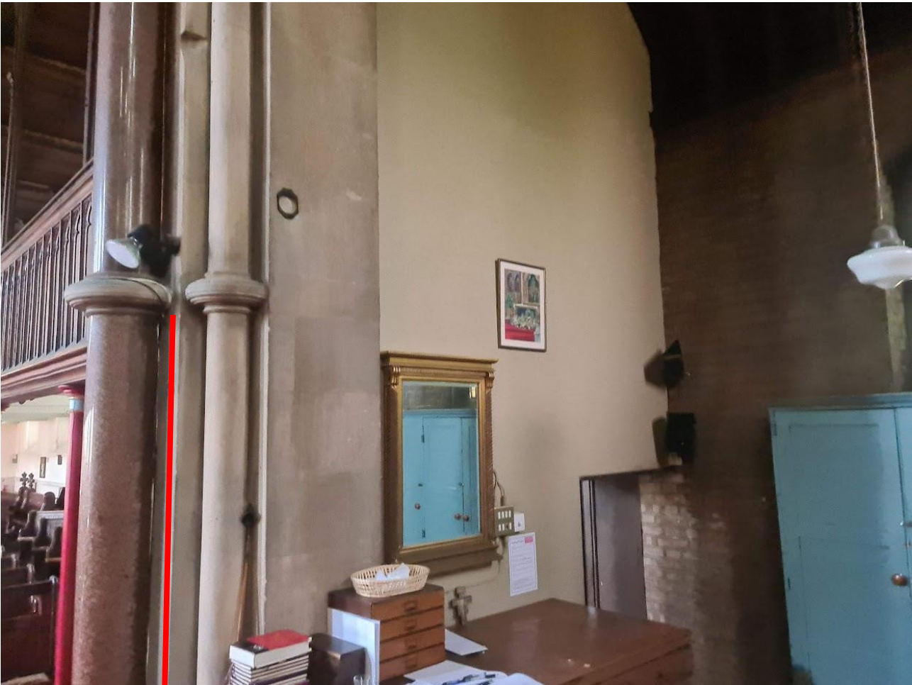
CABLE FOLLOWS DETAIL IN THE CORNER AND EXISTING CABLES FOR MOST THE RUN
