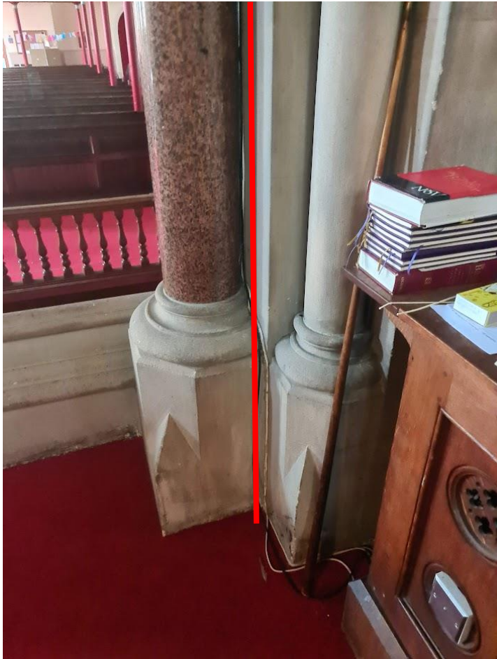
CABLE FOLLOWS DETAIL IN THE CORNER AND EXISTING CABLES FOR MOST THE RUN
